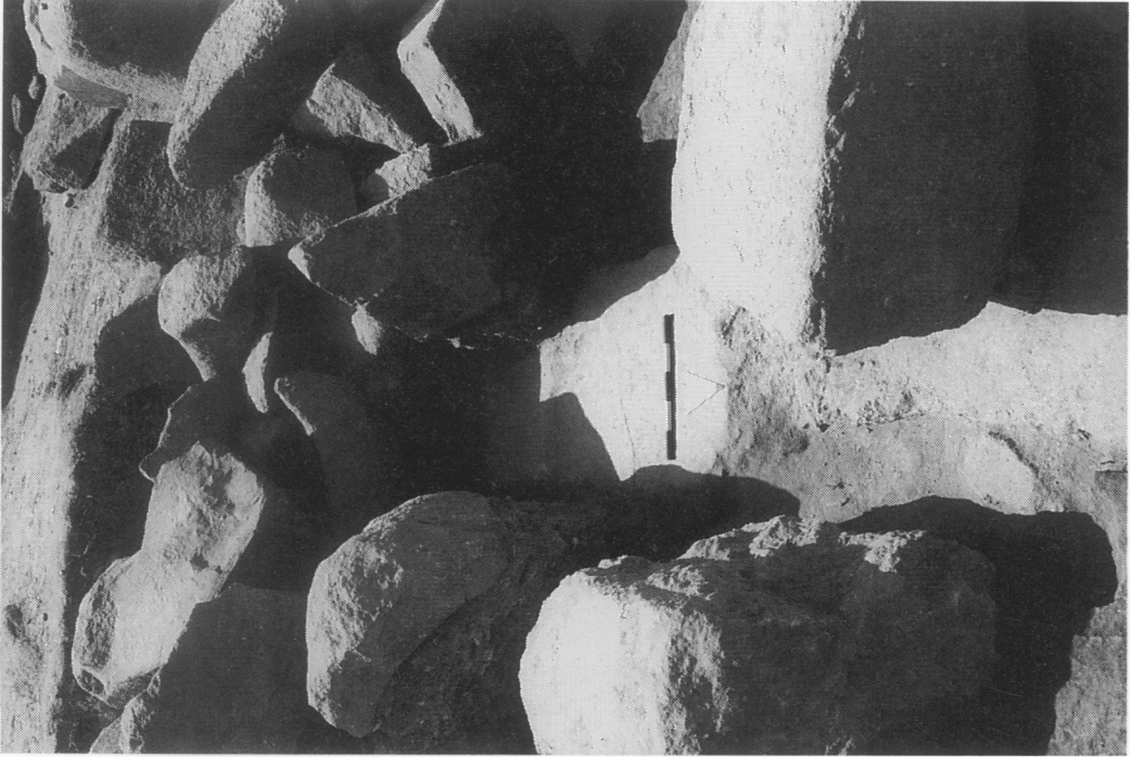
2. Limestone bedding blocks from the west face of the pylon's south tower, seen from the north
